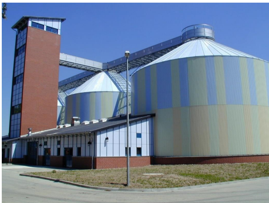
Figure 1. Picture of the three digesters at the WWTP in Steinhof near Braunschweig.
