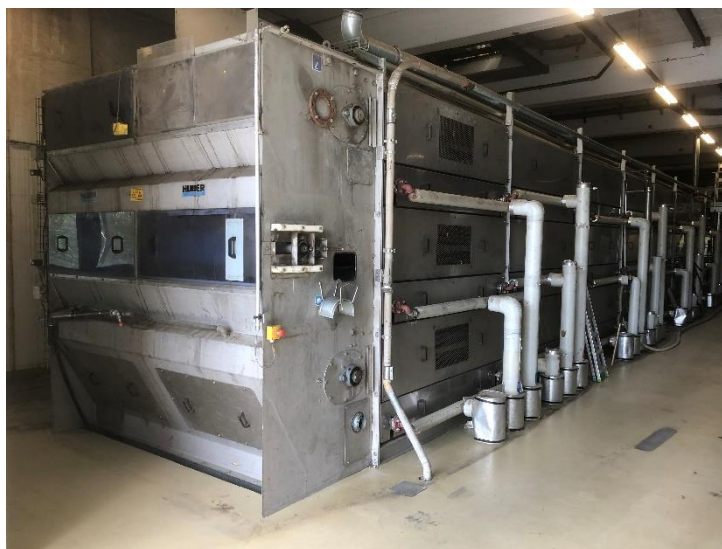
Figure 10. Picture of the drying unit of the sludge treatment stage
